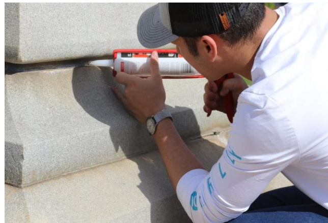
Cleaning and resealing the joint
